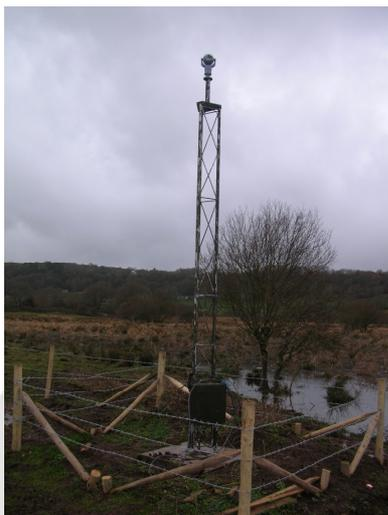
The main camera was installed on a mast which at 4.5 metres tall was in keeping with the height of the surrounding trees. The mast was also camouflaged to allow it to blend in with the surrounding area. The WWC team decided to erect a fence to keep the Water Buffalo from getting too close.
